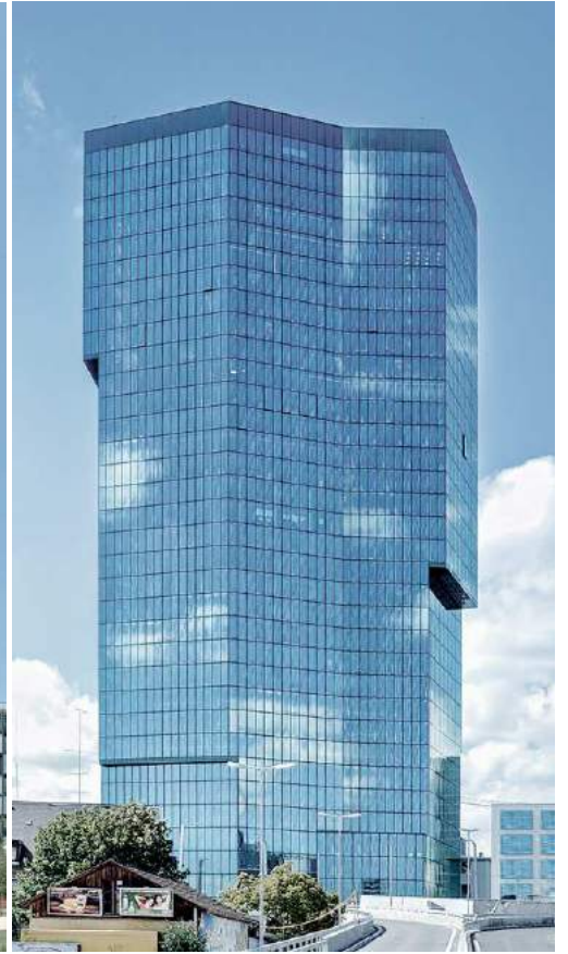
Prime Tower, Zurich Switzerland 126 m
