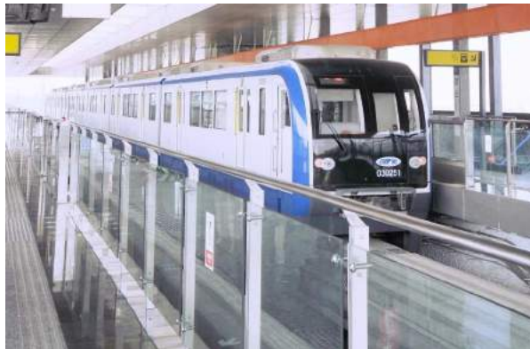
Chongqing Rail Transit, Line 3 Chongqing China
