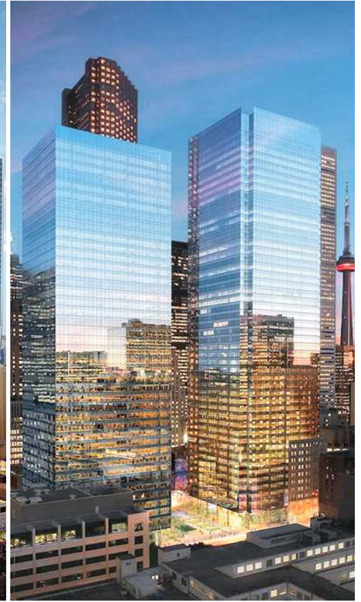
Bay Adelaide East Tower & Podium Toronto, Canada 196 m
